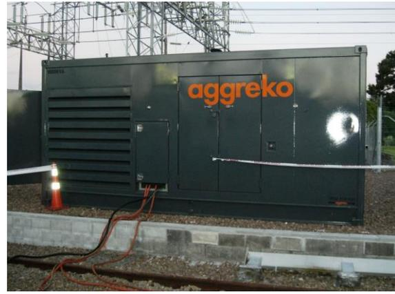
**Fig. 25** Diesel aggregate as source for the resonance test set
