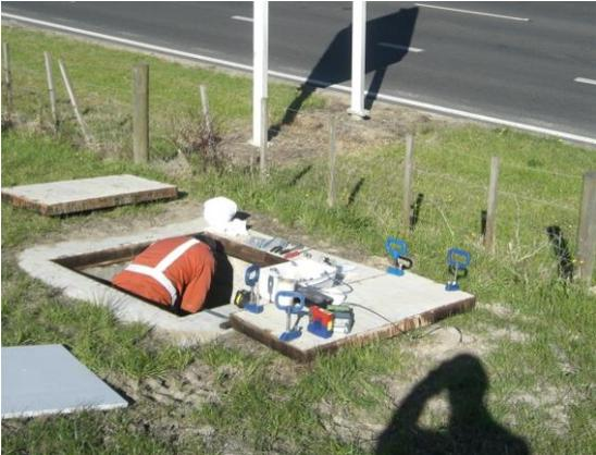
*Fig. 22 Link box close to the highway*
