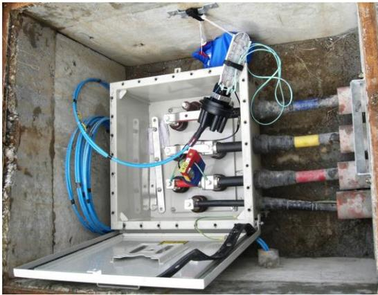
**Fig. 24** Link box for cable grounding with installed HFCT and MPD600 (in the blue bag)
