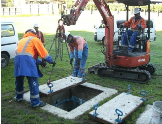
*Fig. 21 Opening of the lids of a link box*
