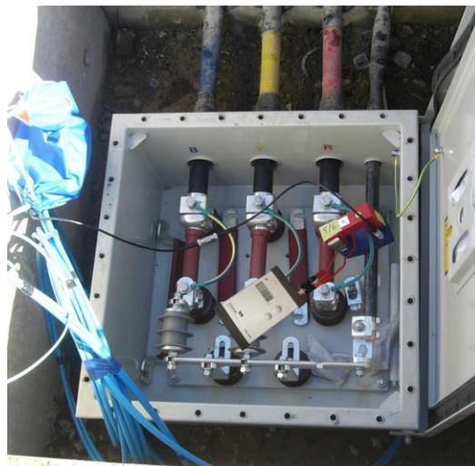
*Fig. 12 Performance check of a HFCT in a link box*
