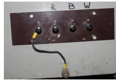
Fig. 2. Secondary terminal box
