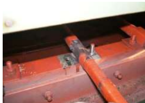
Figure 21 PD source at the conductor to the star point
